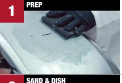
Clean front and back with **Scuff & Clean** and damp, gray scuff pad. Rinse with water and dry or wipe with a clean, damp cloth until removed. Clean front and back with **SEM Solve, Plastic & Leather Prep** or **XXX Universal Surface Cleaner**. Wipe clean in one direction with dry, lint-free cloth.
